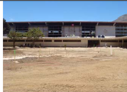
Forecourt during construction
